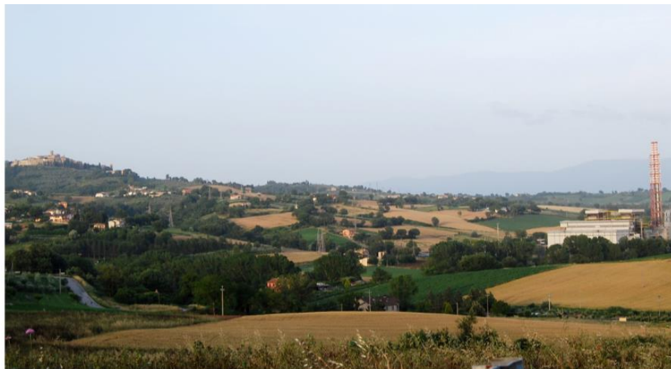
View of the power station (right side of the picture) and of the historic centre of Gualdo Cattaneo (left side)
